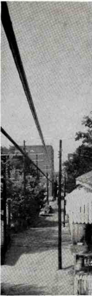
THIS coaxial cable is strung on Southwestern Bell poles.
